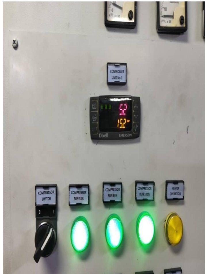
Low Pressure Alarm System After Repairs By Medaan Team
